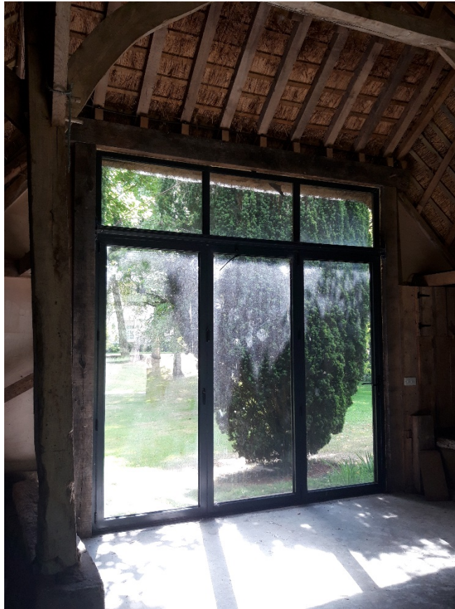
Internal view of South elevation, August 2020
