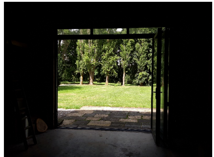
Above and below: Doors in North elevation, August 2020
