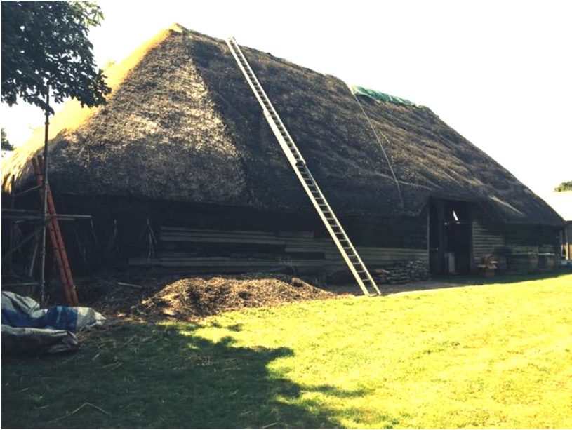
Above: North elevation during re-thatching c.2014, prior to doors being inserted.
